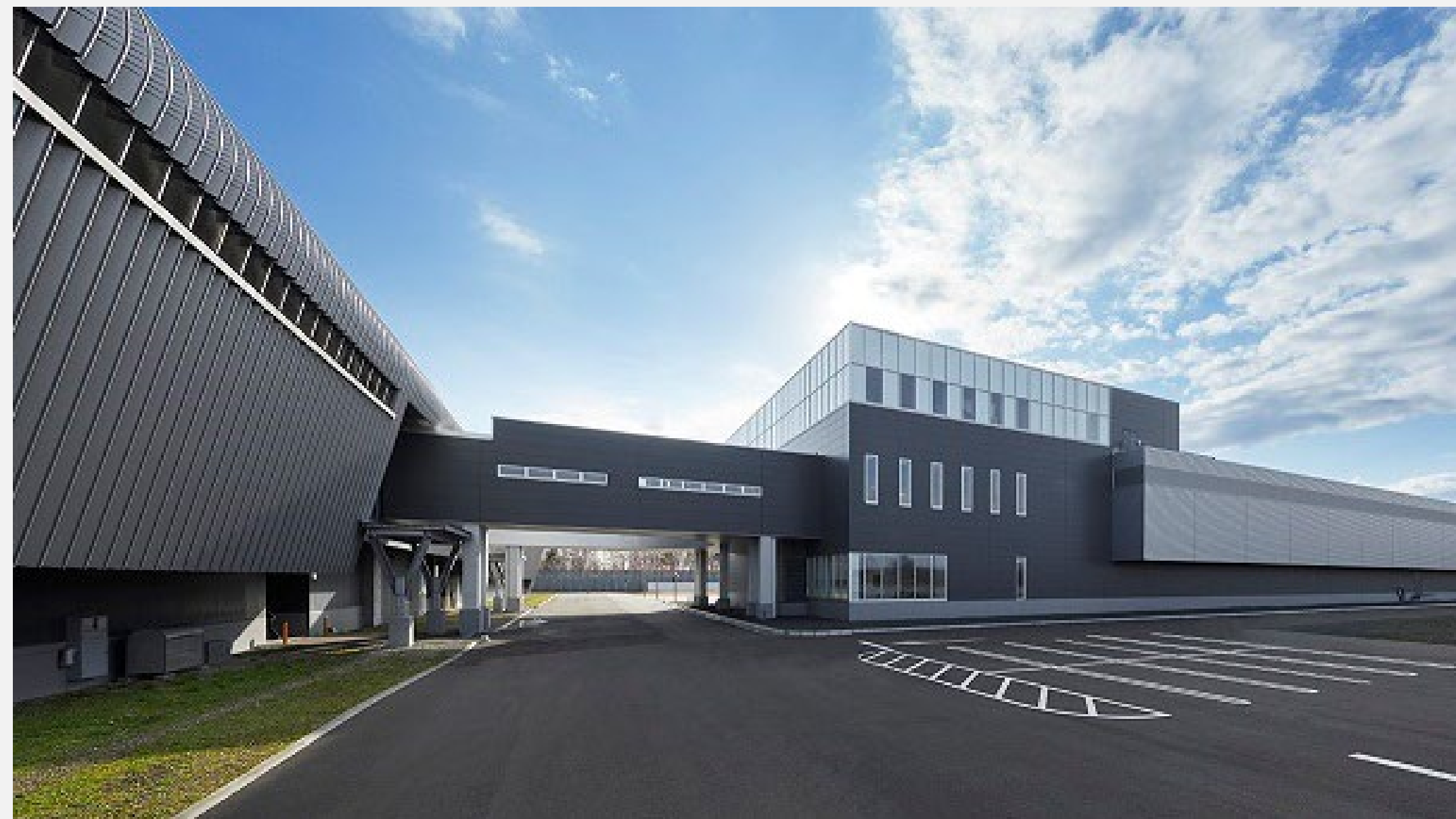
Appearance of Ishikari Data Center (front: Building 3, left: Buildings 1 and 2)
