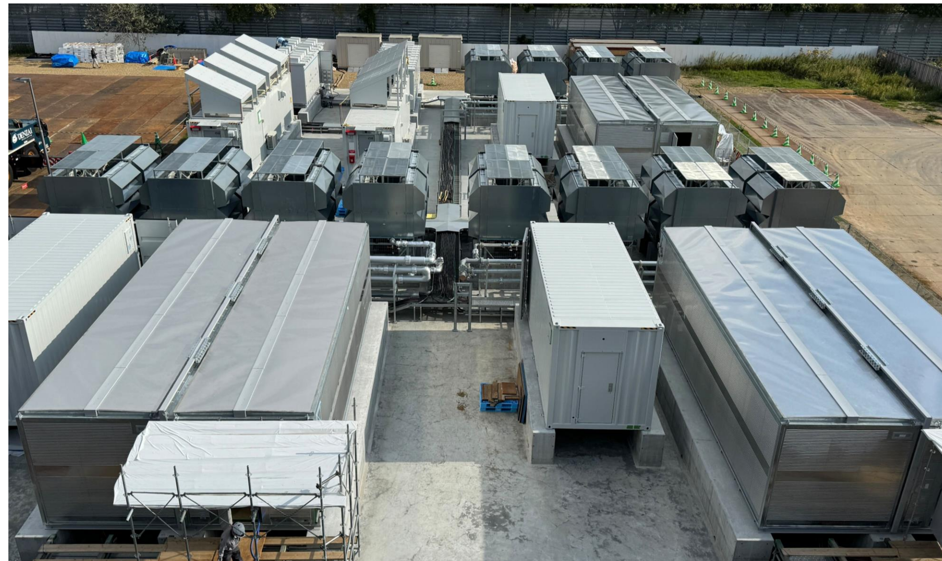
Container-type data centers under construction on the site of Ishikari Data Center
