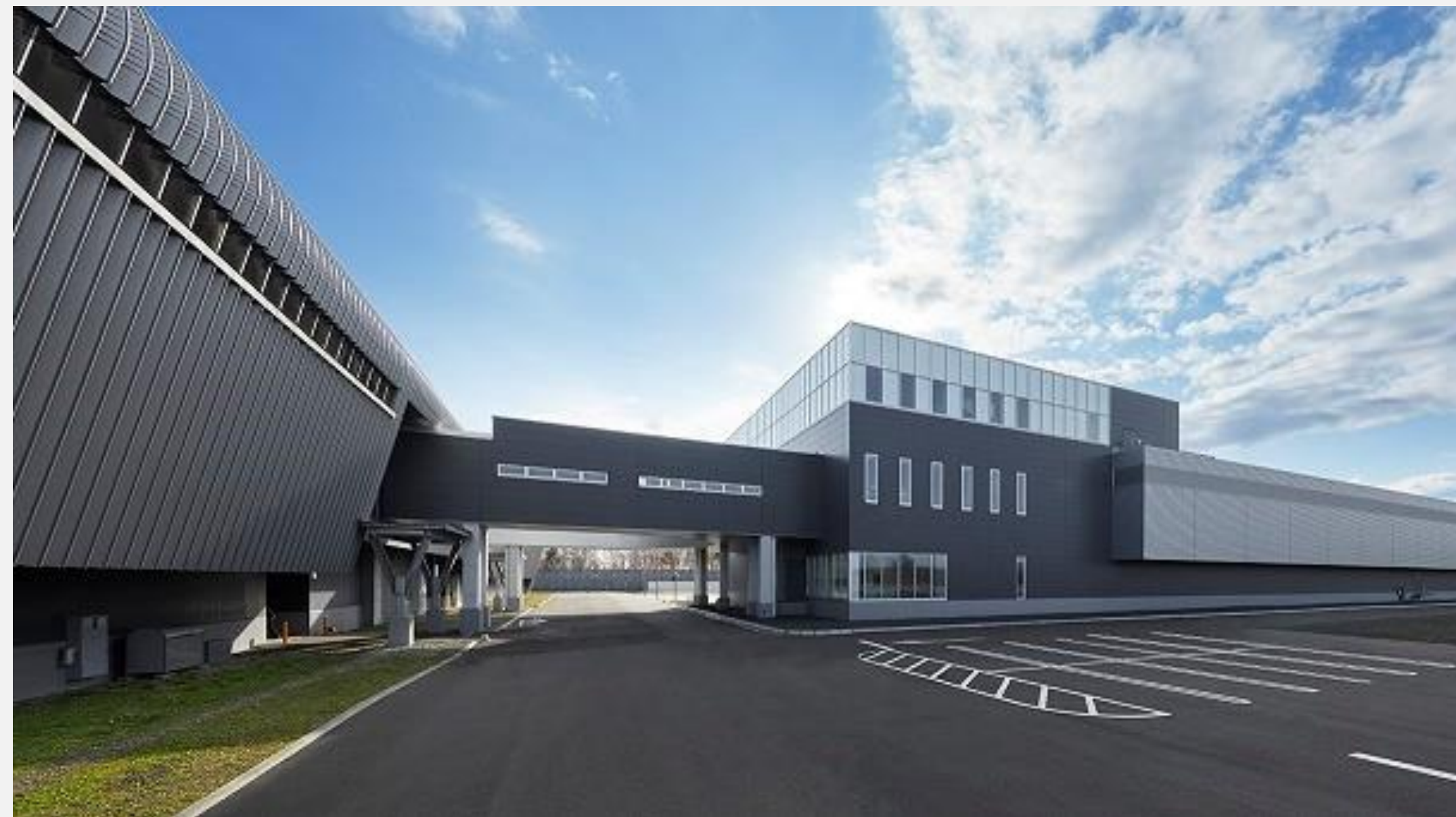
Appearance of Ishikari Data Center (front: Building 3, left: Buildings 1 and 2)
